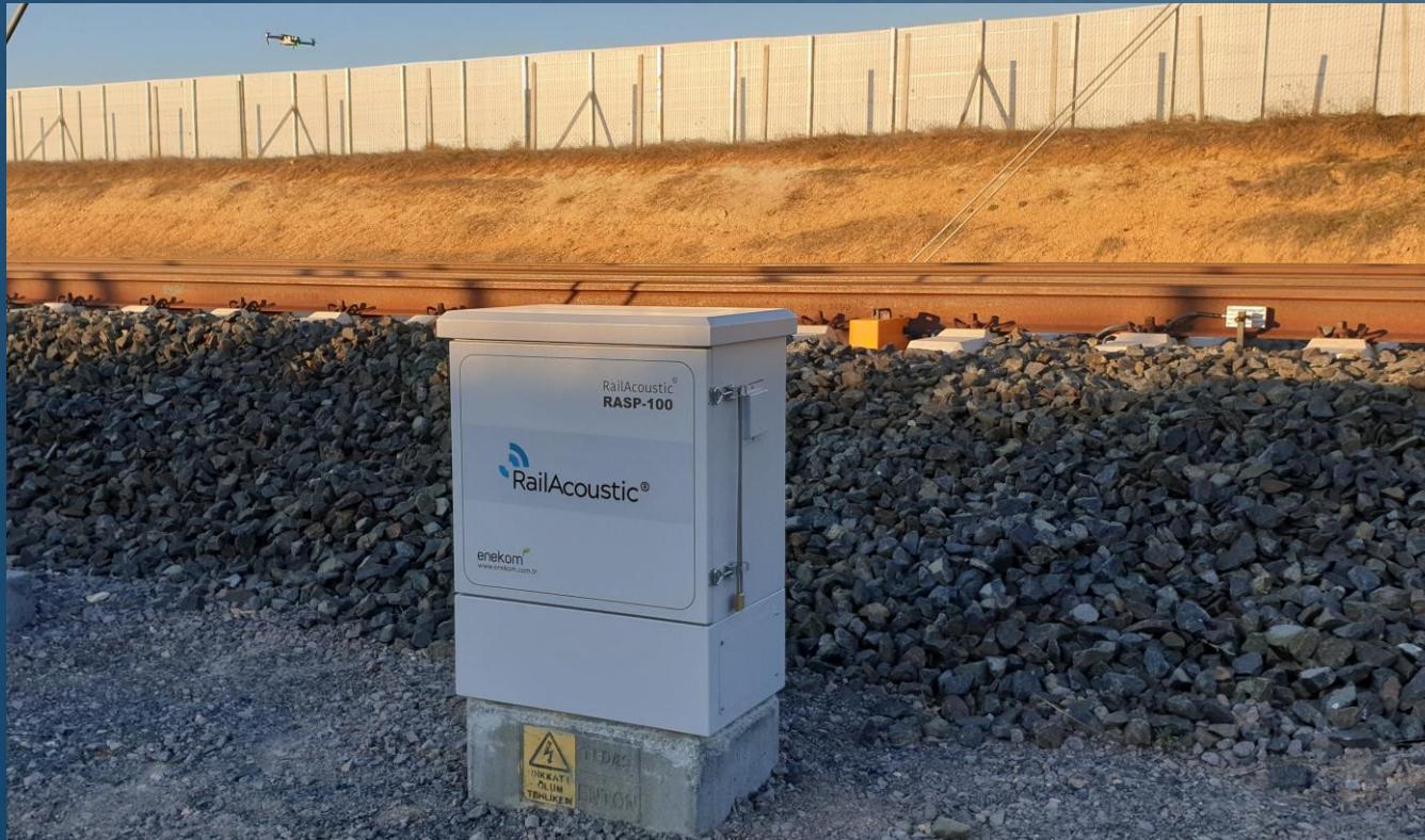
RASP100 Track Signal Processor and Communication Cabinet
