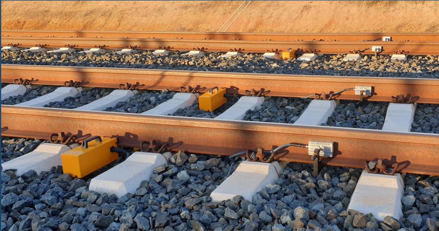
RAG100 and RAR100 Modules Installed on to the Rails
