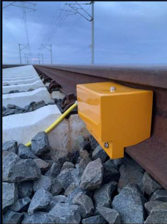
RAG and RAR Modules Installed on to the Rails
