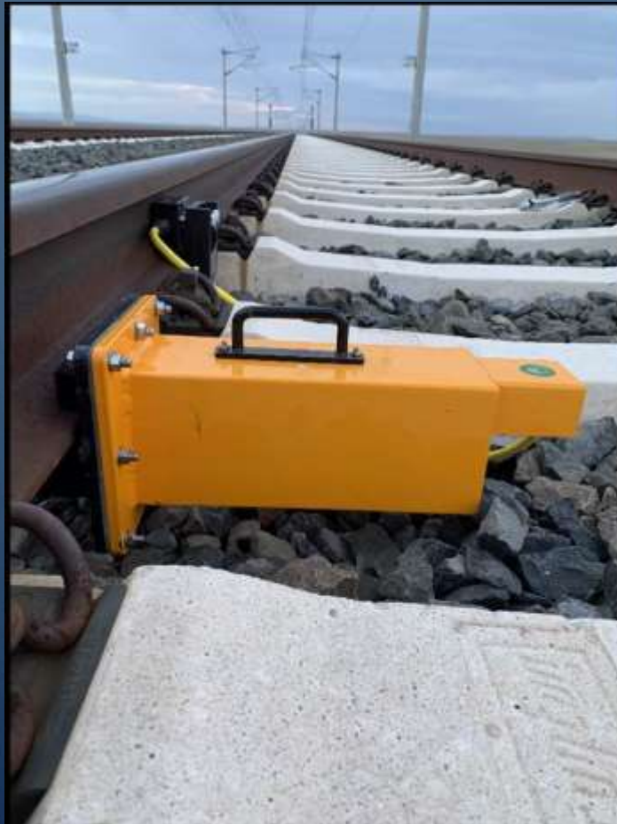
RAG and RAR Modules Installed on to the Rails
